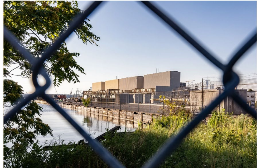
The Gowanus Generating Station in Brooklyn is one of the “peaker” plants targeted by pollution controls. | Ken Schles
